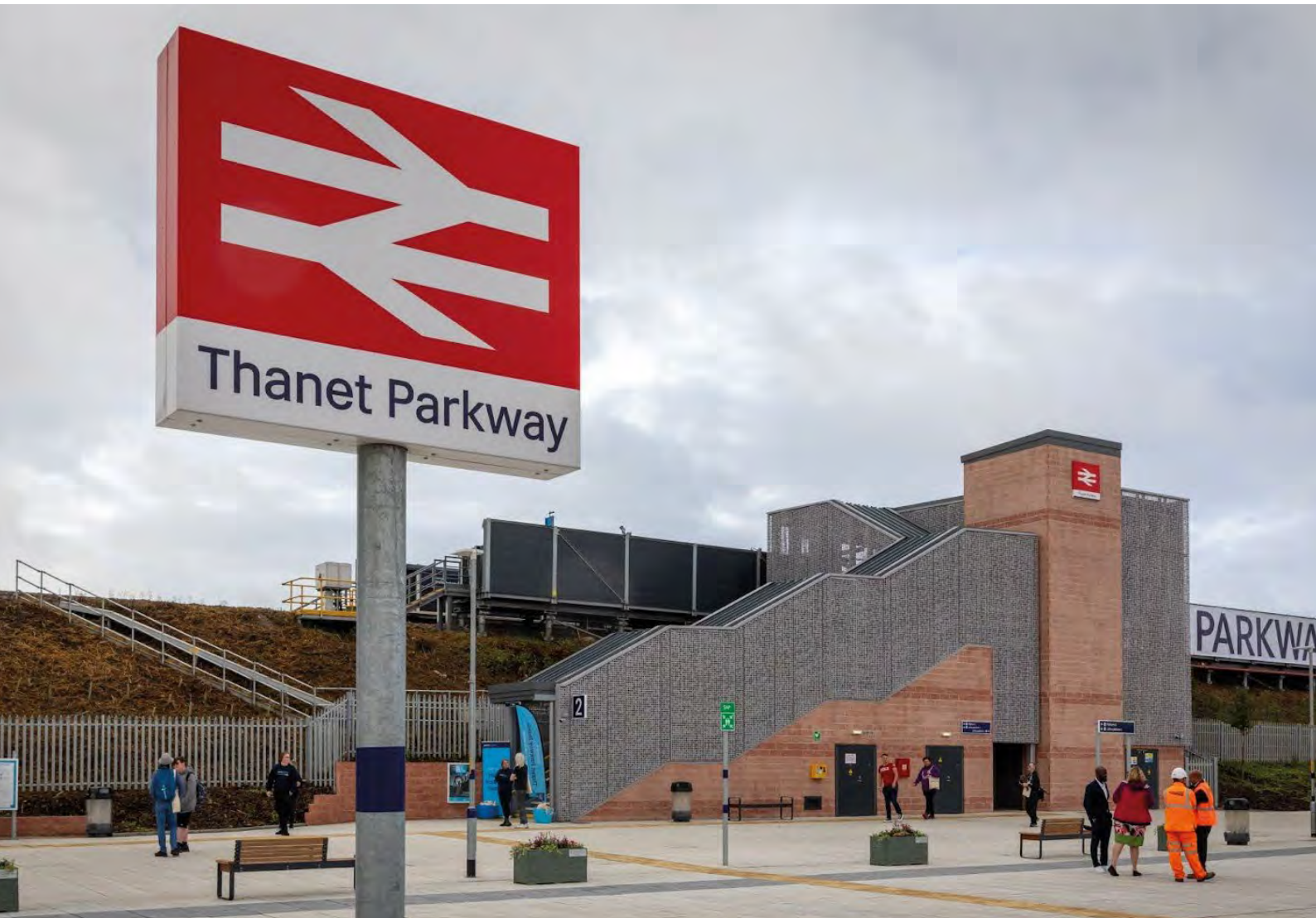
Thanet Parkway rail station.
