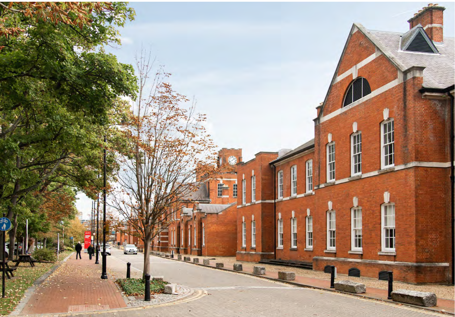
Revival of Chatham Dockyard, University of Kent.
